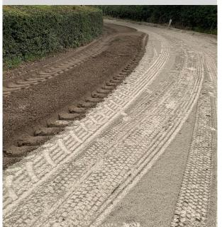
Milestone Infrastructure and their partner Stabilised Pavements Limited carried out the scheme for Oxfordshire, recycling the existing carriageway to re-engineer and rejuvenate the road. This involves pulverising the existing carriageway in-situ and then mixing with a small volume of foamed bitumen and cementitious powder to create a new strengthened carriageway in a cost effective and sustainable manner.
