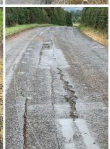
North of Berrick Salome in rural Oxfordshire an unnamed road approximately 2km in length required structural maintenance after its shape and surface was being impacted by some deeper cracking in the foundation layers.
